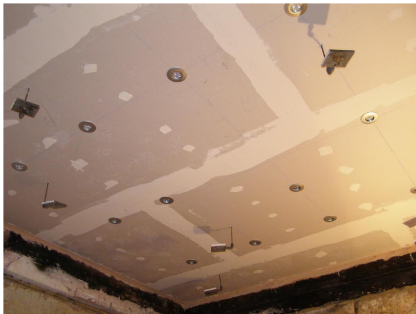
Plate 2 Exposed face of test construction before test showing downlights installed.
