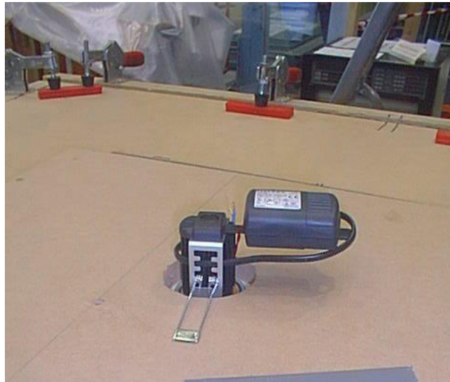
Figure A3. Above the ceiling part of the Halers H2 down light fitting
